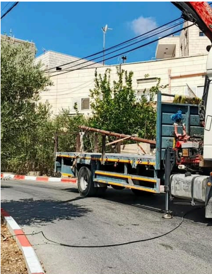
Removing disused poles from the city's streets.
